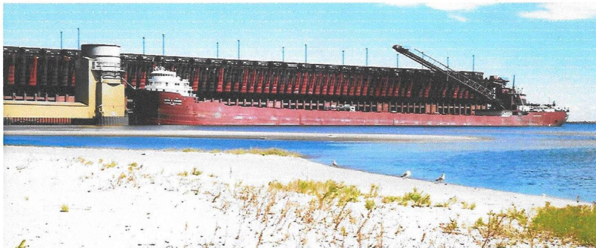
The LS&I railroad docks in Marquette, with the last addition, an unloading hopper for self-unloaders to discharge coal and limestone. The "Kaye E. Barker", above has both a bow and a stern thruster to aid in maneuvering.
