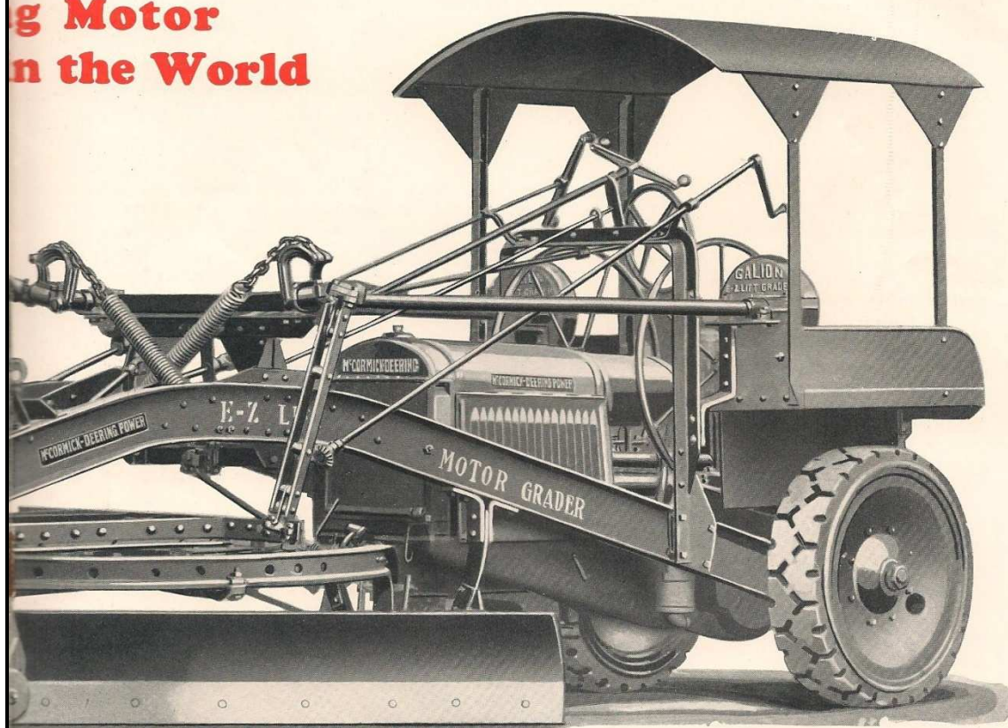
Galion McCormick-Deering E-Z Lift Motor Patrol Grader Complete with Rubber Tired Wheels, Cab and Scarifier
