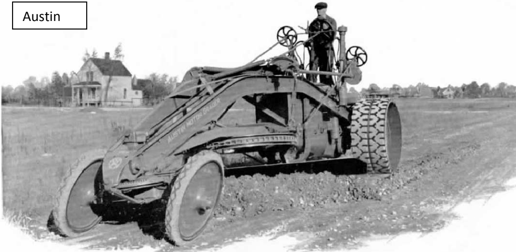
The 15-30 Model maintaining a hard, rough road. The leaning front wheels hold the machine to a straight course in spite of the heavy load on the blade.
